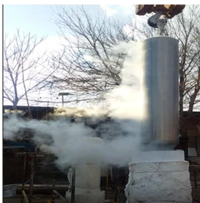
Fig. 6 Transferring vessels 2 of liquid nitrogen for shrink Fit
