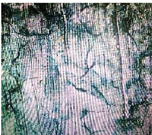
Fig. 6 Cracks formed on surface of the specimen at 50 mm displacement of punch in tube flattening test
